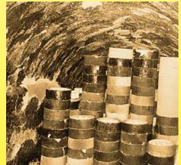
Traditional Chinese Dragon oven (龙窑 Long Yao), feeding mouth and filling method with electric porcelains (private collection)
